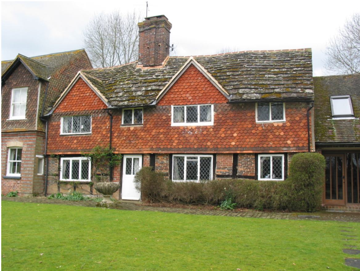
Fig 53 Coldharbour Farm, Cranleigh, 1683 , showing its forward-facing gables, big central chimney, and Horsham stone roof.
