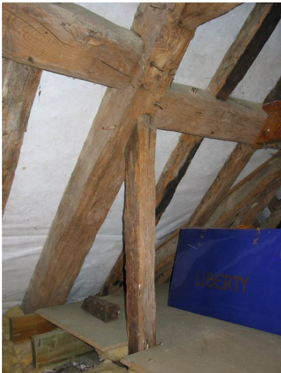
Fig 54 Coldharbour Farm, Cranleigh, 1683 , staggered-butt-purlin roof structure. If the mortices were in line, they would weaken the structure. It is a good sign of a late 17th century house, although there are occasional earlier examples.
