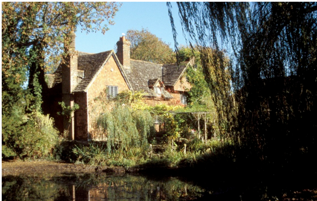
Fig 29 Taylors, Capel , has pleasures of a different kind. It is extraordinarily picturesque and needed a combination of archaeology and dendrochronology to unravel its history: west wing (left), 1345; centre part, 1467m; east wing, 1642m. The Horsham stone roof and tile-hanging are very 'Surrey'.
