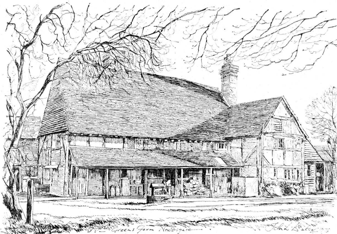
Fig 21 Greens Farm, Newdigate, 1309 , with a soaring roof and giant crown posts - the earliest such posts dated by the Project. The wing to the right is newer, as is the chimney and pentice roof along the front. Drawing by John L Baker, reproduced courtesy of the Surrey Advertiser .
