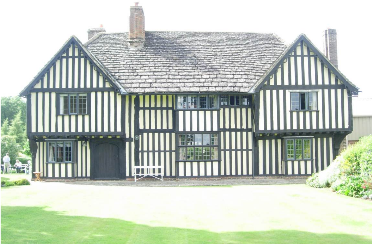
Fig 22 Brewerstreet Farmhouse, Bletchingley, 1491 , a variant Wealden house of unusual riches and design. Note the forward-facing gables, full-height close studding, ‘Horsham’ stone roof, ornamental barge boards and arched doorhead. The farmhouse was rescued from dilapidation by the owner. Photograph by Patrick Moyle.
