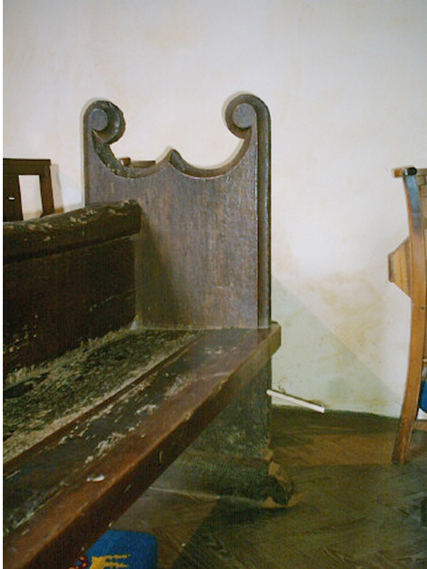
Fig 76 Dunsfold church pews dated to 1418 (modal). Simon Jenkins (2000, 673) suggested that they could be contemporary with the 13th century church, which could make them as old as any in England. This is now shown not to be so, but they are still ancient and of much interest. The bench-ends have deep cusps ending in knobs with holes for carrying lighted tapers. Six cores were taken from inconspicuous places. The dowel that can be seen at the bottom right shows one such place. It is good practice to mark each position photographically in this way as a record of from where they were taken.
