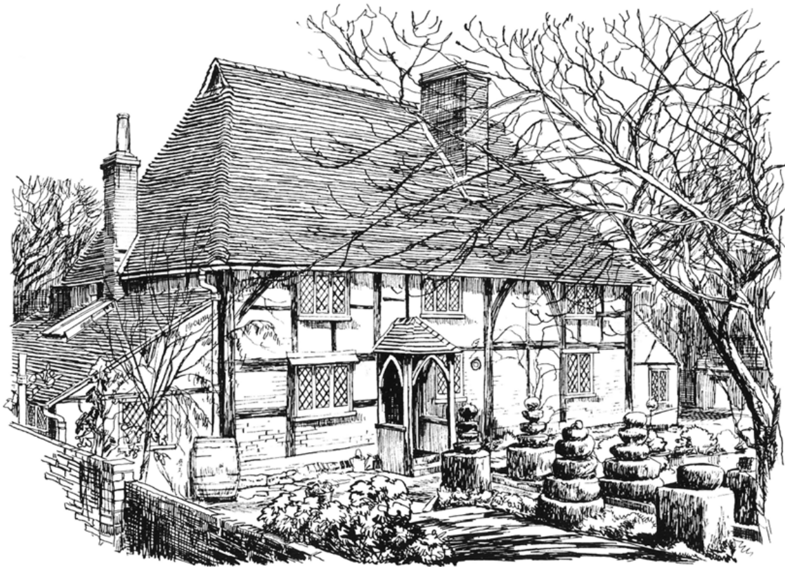
Fig 8 The Old Cottage, West Horsley , is a medieval open-hall house with a tall crown-post roof and arch braces in the framing. A combination of dendrochronology and archaeology was needed to understand the building and establish that, while it was built in 1445, the western (left-hand) bay was rebuilt in 1563. Drawing by John L Baker, reproduced courtesy of the Surrey Advertiser .
