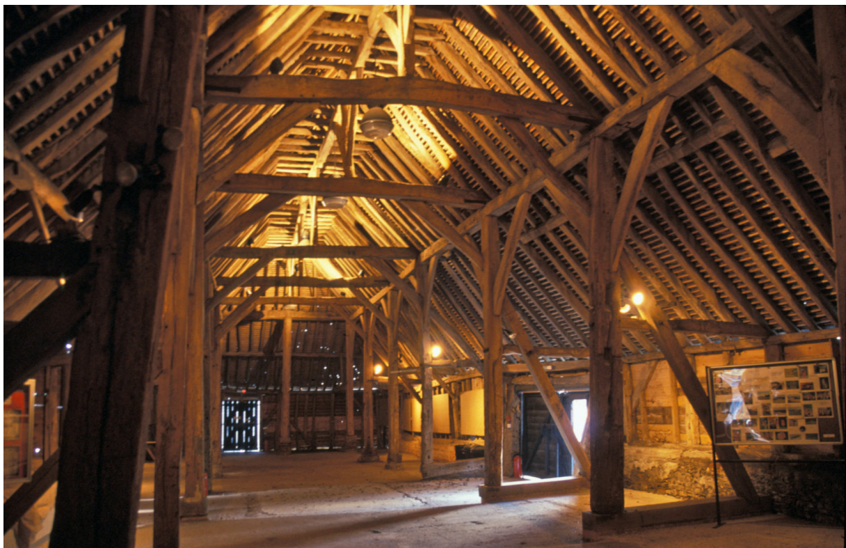
Fig 15 Wanborough Great Barn, 1389 , a spectacular crown-post building often open to the public (contact Guildford Museum for opening times).
