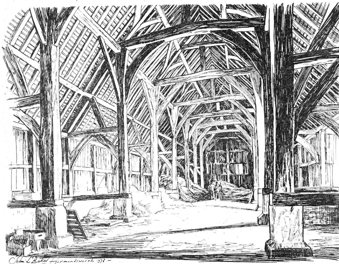
Fig 47 The Great Barn, Harmondsworth, 1426 , is a magnificent barn linked to William of Wykeham, Bishop of Winchester (Impey 2017, 13). The structure is pioneering, with single central crown struts, forming 'T' shapes with their collars in the roof. The struts are like crown posts, but there is no central collar purlin joining their tops along the length of the building. Instead the collars hold in place side purlins, quite new and much more efficient. Drawing by John L Baker, reproduced courtesy of the Surrey Advertiser .
