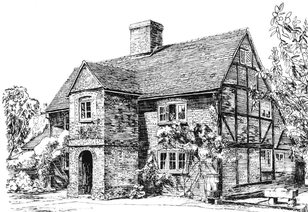
Fig 11 Whites Farm, Worplesdon , is a central-chimney house with some timber framing remaining to the side. There is a fine two-storey porch of a kind sometimes seen in Surrey (see also Frosbury Farmhouse, frontispiece). The date of 1670sto (see below) can be seen on the front of the porch, picked out in flints. There is evidence in the roof that the porch is coeval with the main house, so the date applies equally to both. Not visible from the front is an older part to the rear, probably 16th century. Drawing by John L Baker, reproduced courtesy of the Surrey Advertiser .
