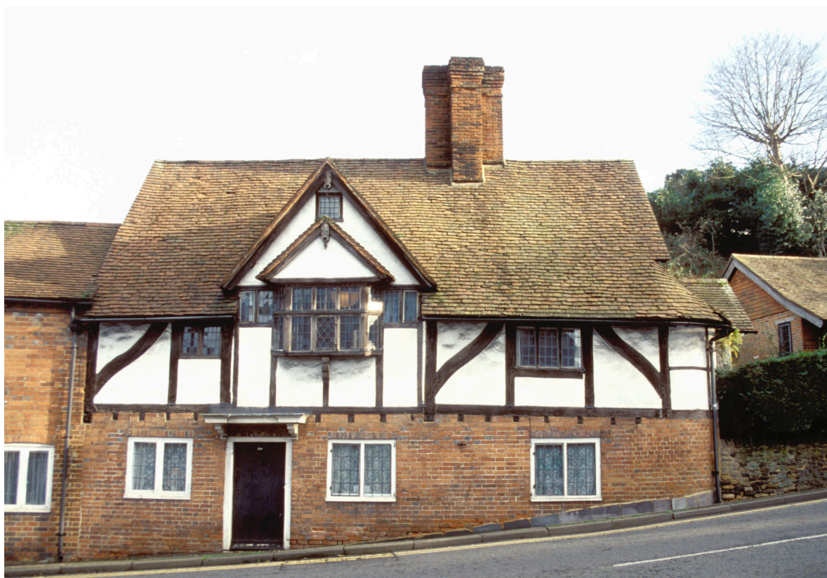
Fig 46 11 Bridge Square, Farnham, 1476 , is a well-disguised Wealden-style house, the jetties having been under-built and the recessed centre filled in. A forward-facing gable was added, with a remarkably-carved oriel window, now very much a feature of the house. It is unusual in a number of ways: a half-floored hall (discussed above); attractive ogee braces; and a roof of clasped-purlin construction – at this date elsewhere in Surrey it would have crown posts.
