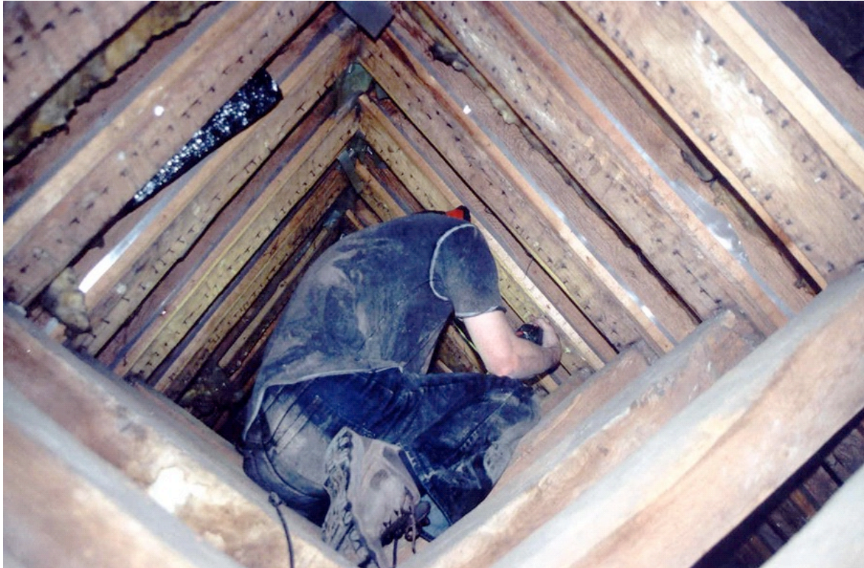
Fig 4 Bishop's Camera, Farnham Castle (dated 1381). Andy Moir working above the scissor bracing in the roof of the. Sometimes agility is needed as well as dendrochronology.
