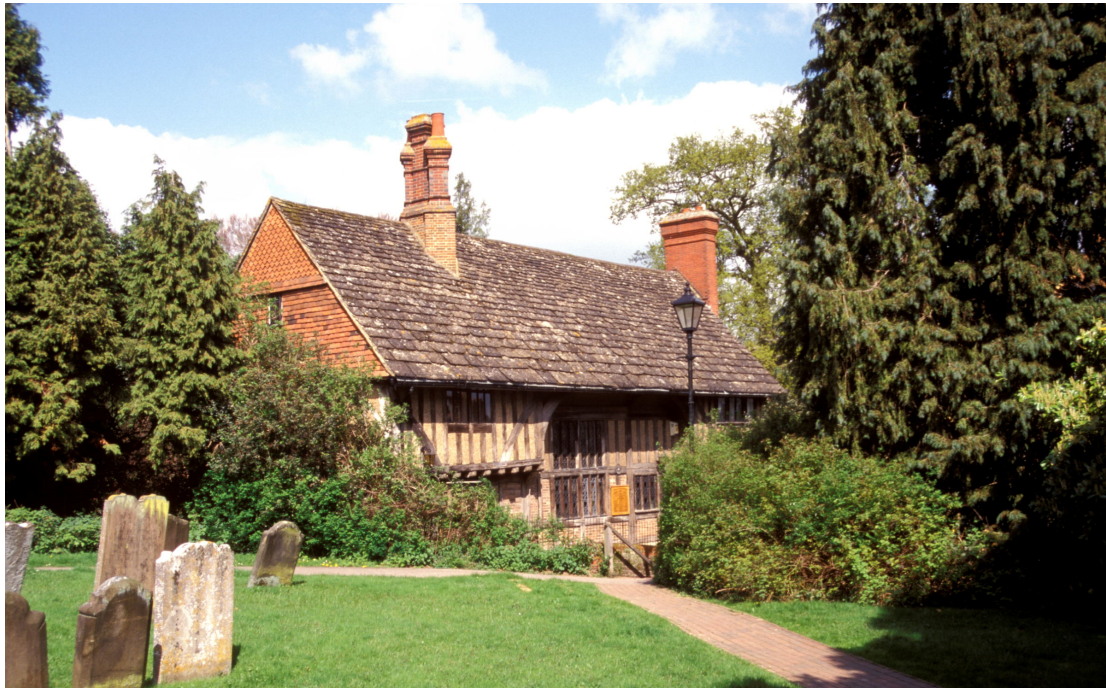
Fig 28 The Guest House, Lingfield, 1474 , is a stunning example of the pleasures of traditional timber-framed buildings. It is in the Wealden style, with jetties, a bridged-over centre, close studding, and a Horsham stone roof. It may have been the hospitium for a monastic college. The interior is just as beautiful, with a rich open truss. It is a public library, so open to all. It has been restored, but the masterful carpentry shines through.
