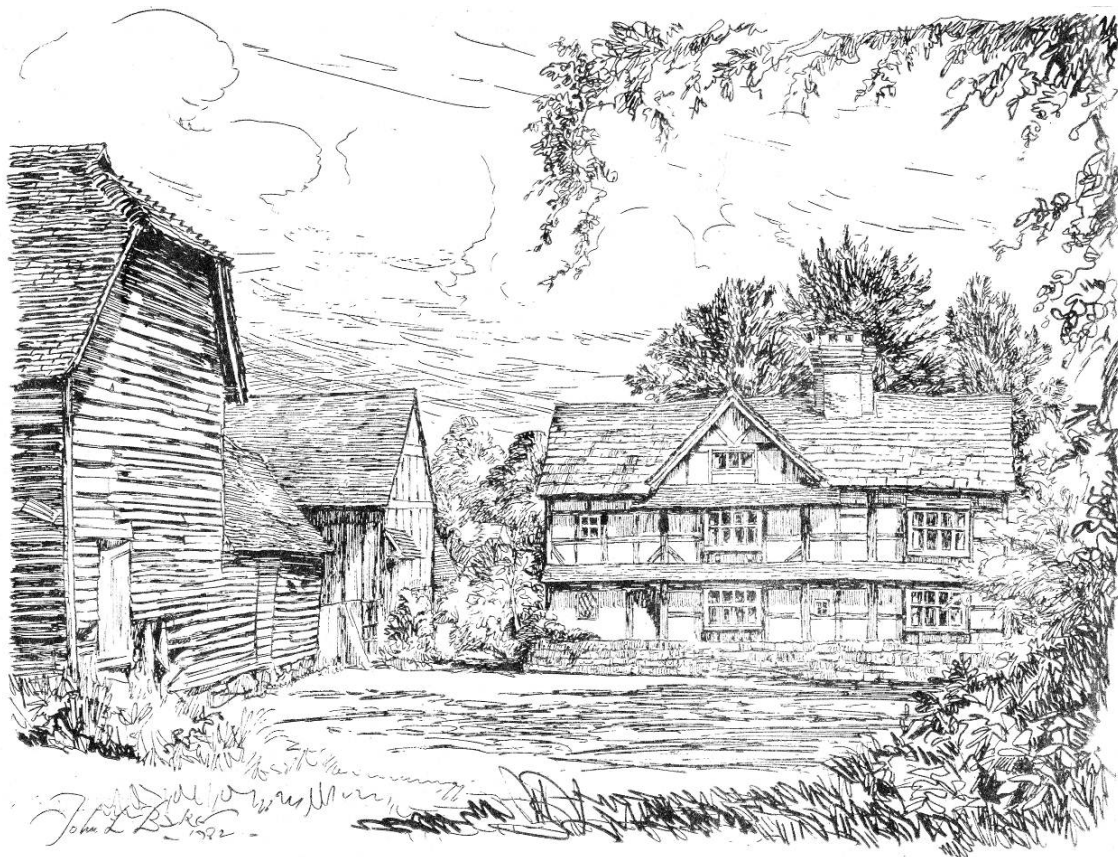
Fig 27 Volvens, near Ockley (Abinger parish) 1623. A textbook example of a higher-status 17th century house, with a central chimney, a forward-facing gable, small square panels with short straight braces, oriel windows and a pentice roof. Drawing by John L. Baker, reproduced courtesy of the Surrey Advertiser .
