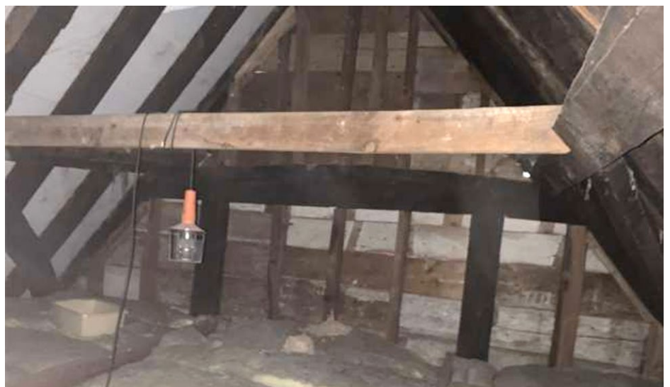
Photo looking to truss Y'Y showing smoke blackening
