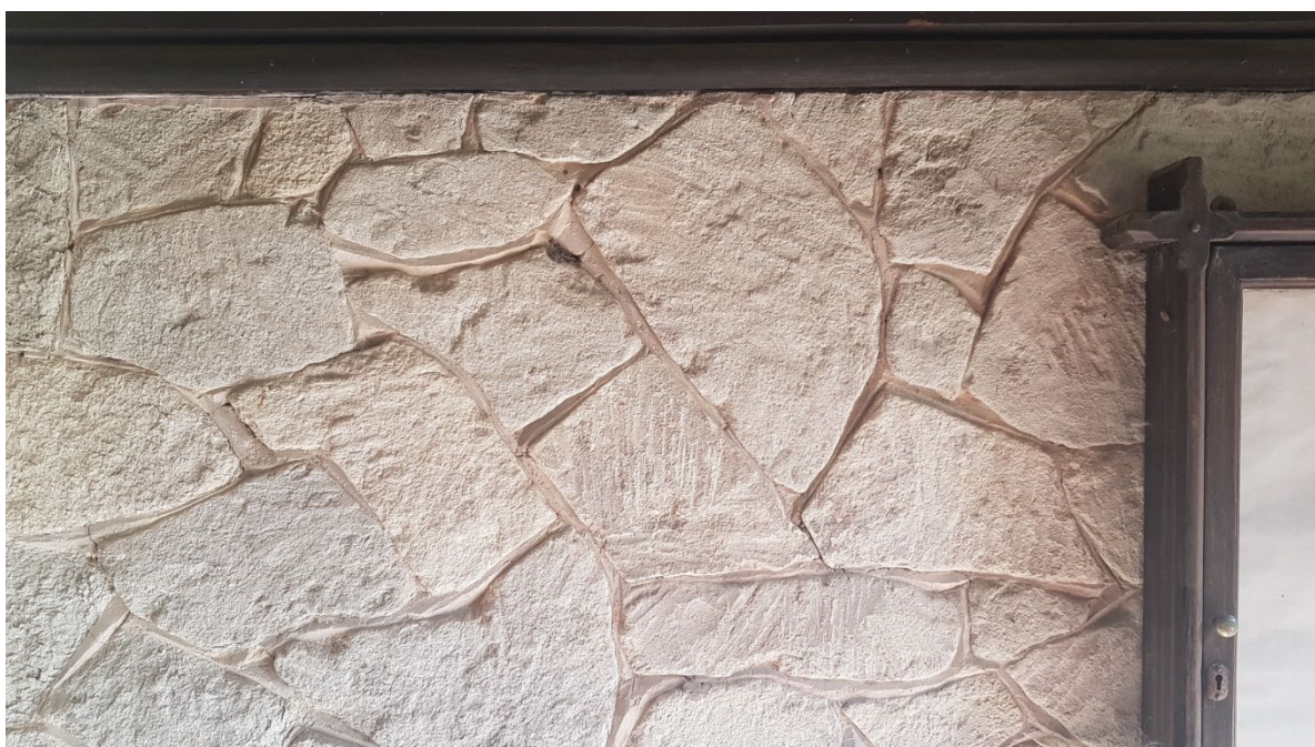
Nineteenth Century “crazy paving” stonework
