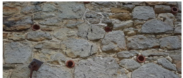
Detail of land drains used as ventilation
