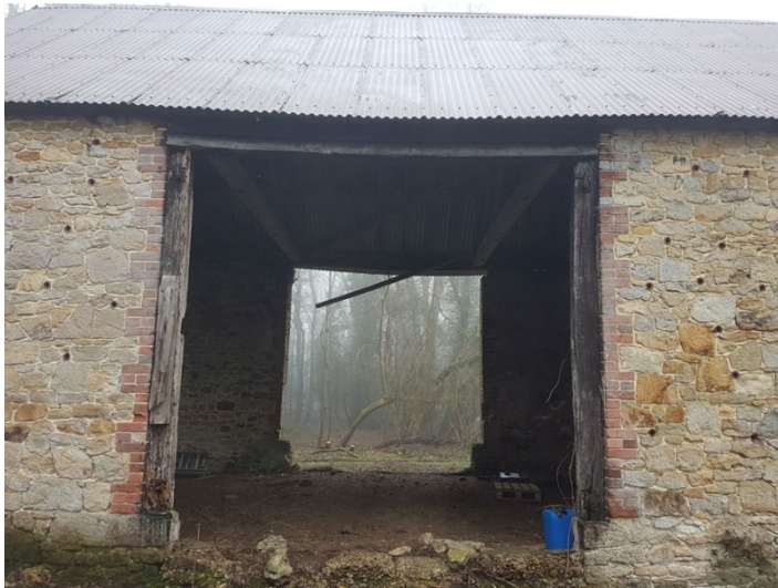
South elevation of the barn showing the round land drains to allow ventilation
